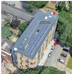
Twelve Acres House: A newer block. Opportunity for low carbon heat, fabric measures could be upgraded if surveys find this to be necessary.
