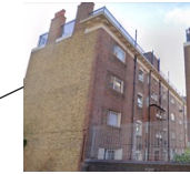
Avondale House : A priority block. Slightly more complex façade but opportunities for window replacements, some wall insulation, roof insulation and PV
