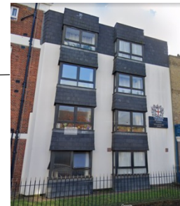
Donnelly House House: a 1980s block but with 40% EPCs at D or below. These are potentially heat pump ready with retrofit opportunities to roof, windows and wall.
